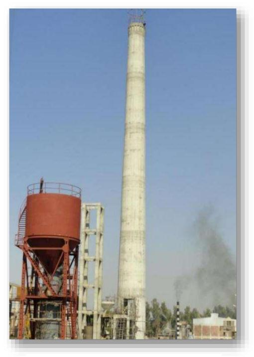
**CLIENT:** NISHAT TEXTILE POWER HOUSE TAPERED STACK WITH 5.0 M LOWER DIA, 3.0M UPPER DIA AND 60.0 M HEIGHT
